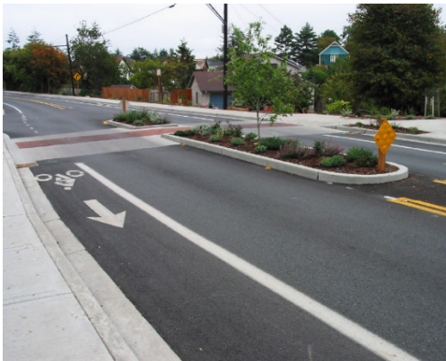
Pedestrian island and bicycle lane traffic calming measures. Photo source: Richard Drdul
