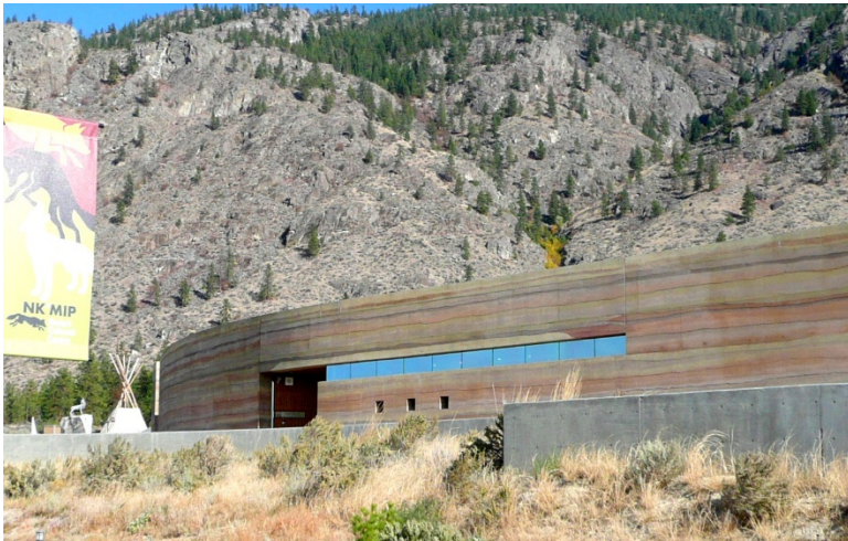
Nk'Mip Desert Culture Centre in British Columbia. Photo source: Architect21c
