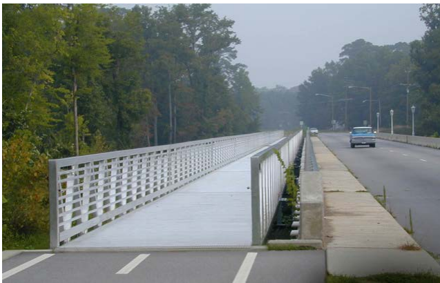
Retrofit of an aluminum bridge to an existing highway bridge with inadequate pedestrian facilities. This is typically a less expensive option than widening of an existing bridge. Photo source: MAADI Group
