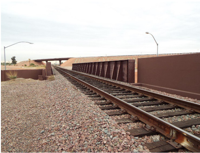
Railroad grade separation from two-lane local highway in Peoria, IL.
