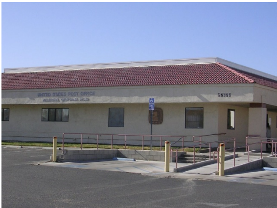
U.S. Post Office in Helendale. Photo source: Panoramio, Scott Vee
