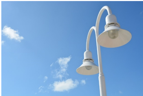
Streetlights aimed downward decrease light pollution and spillover. Photo source: Pixabay, wildkatkca
