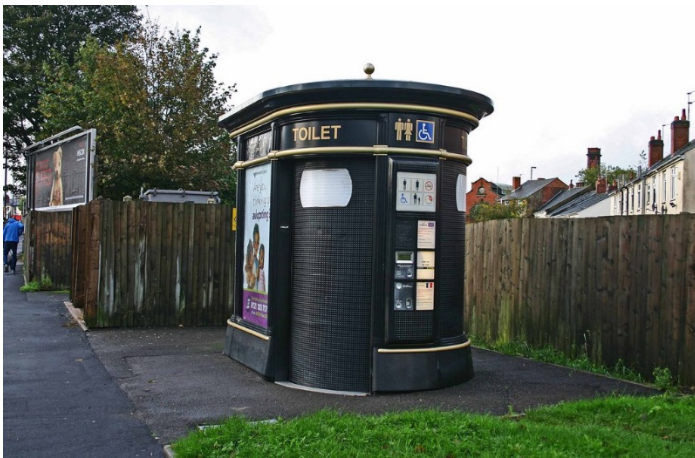
Restrooms accessible to the public. Photo source: P L Chadwick
