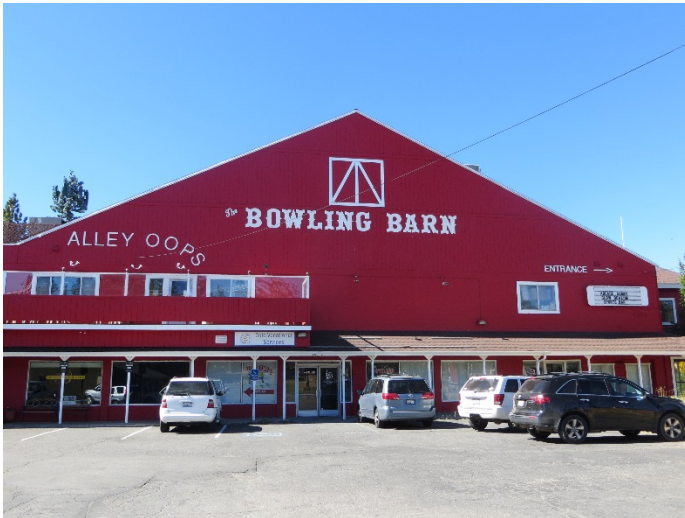
Clean storefront signage improves the overall appearance of commercial structures. Photo source: Michael Baker International
