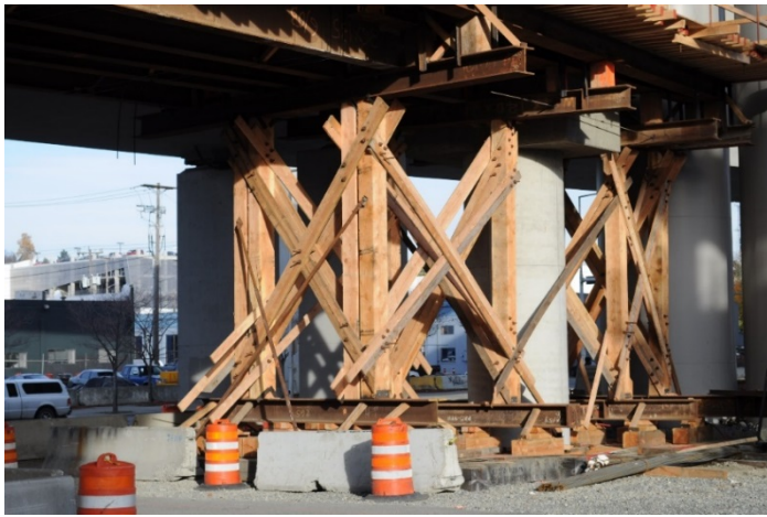
Freeway interchange construction in Seattle, Washington. Photo source: Joe Mabel
