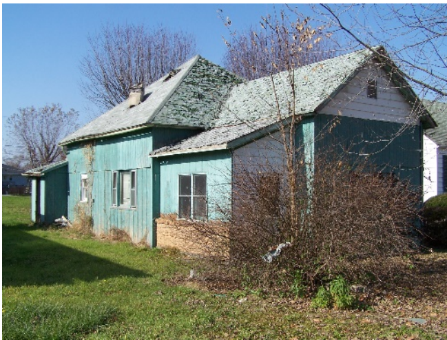
Single family home in need of rehabilitation. Photo source: Valerie Everett
